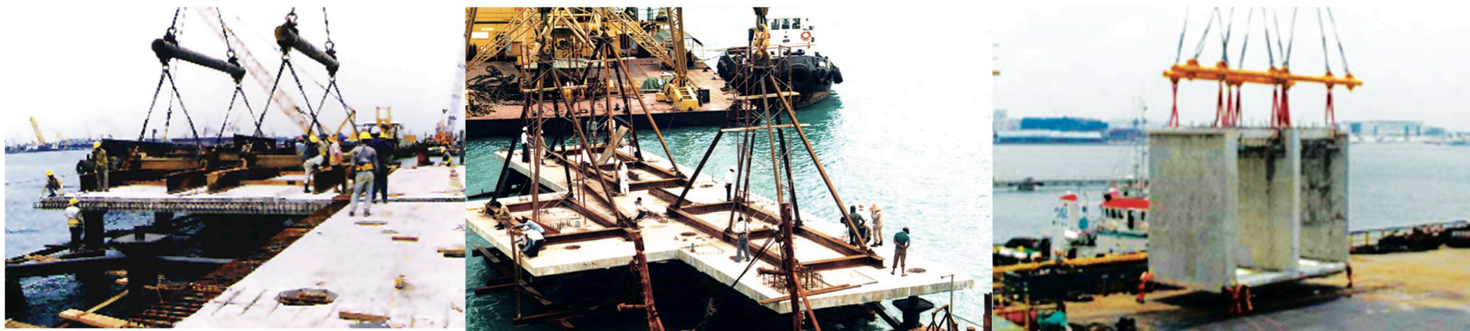
Large Module Precast Flat Slab Construction
