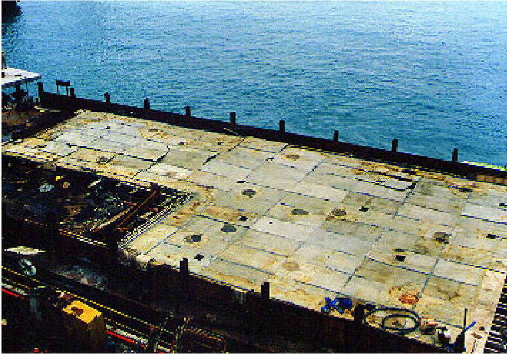
Photo 3 : Formwork for precasting on a pontoon
