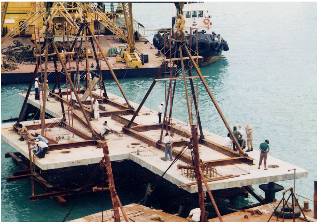
Photo 4 : Lifting an entire deck in one piece(1987)
