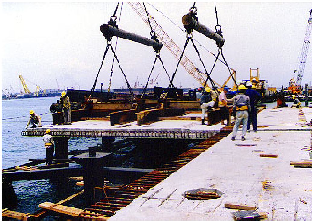
Photo 2 : Thin, lightweight flat slab system
