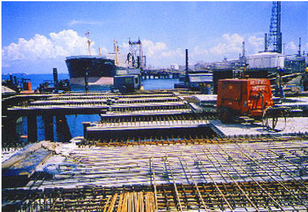
Photo 1 : A conventional precast concrete deck consisting of precast beams and slabs, tied together by in-situ concrete top
