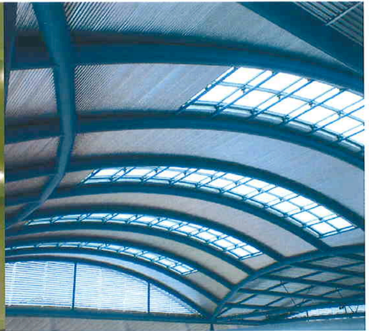
ROOF OVER SWIMMING POOL
