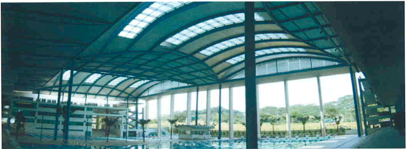
SINGAPORE SPORTS SCHOOL SWIMMING POOL ROOF
